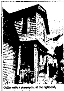
Gutter with a downspout at the right end, coming down the column.
