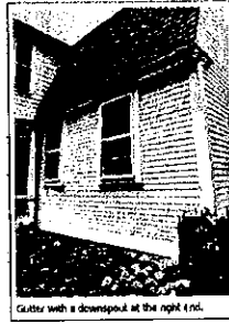
Gutter with a downspout at the right end.
