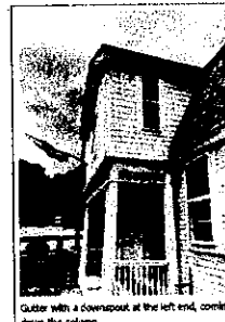
Gutter with a downspout at the left end, coming down the column.
